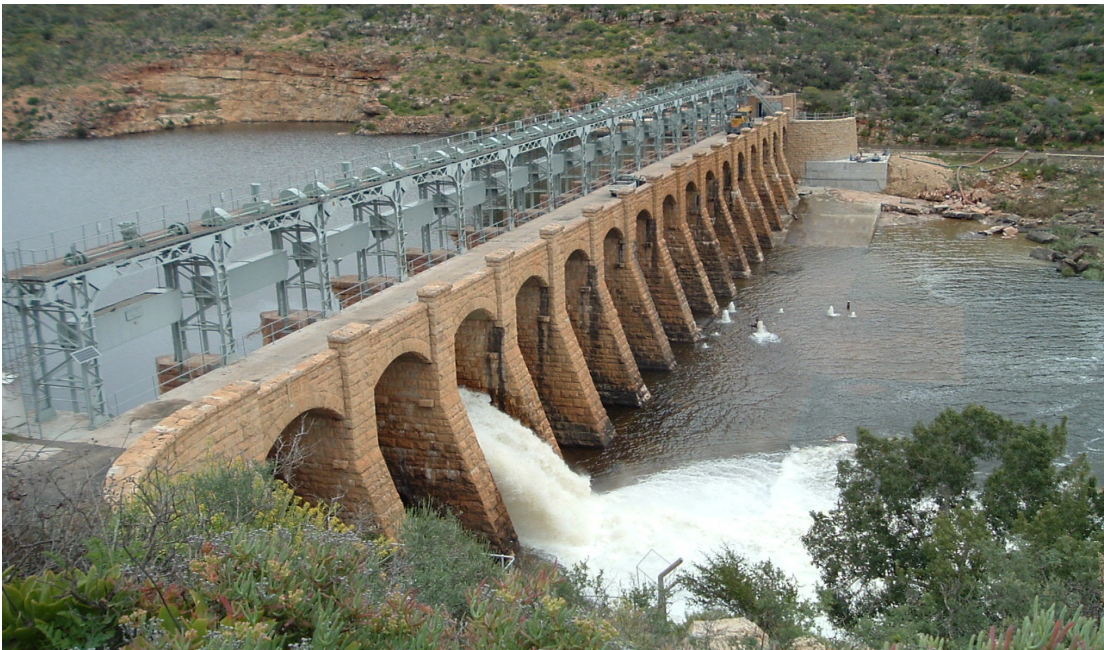
Figure 2.1 The Bulshoek Weir
