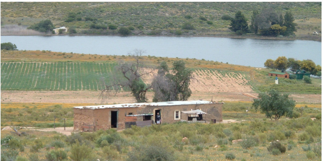
Figure 2.2 Farm worker's house upstream of Bulshoek Weir
